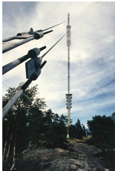
Fig. 14: The parabolics are fixed to the stiff concrete tower
