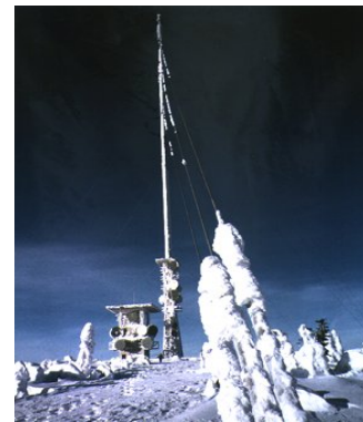
Fig. 3: Atmospheric icing and in combination with wind may be decisive for the design in some locations
