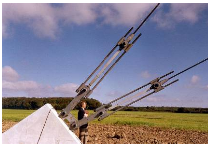
Fig. 15: Guy attachment to foundation with tension system
