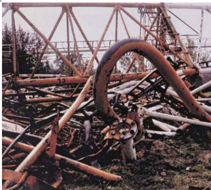
Fig. 1: The tallest mast in the World, the 648 m high long wave mast in Konstantynow, Poland collapsed in 1991
