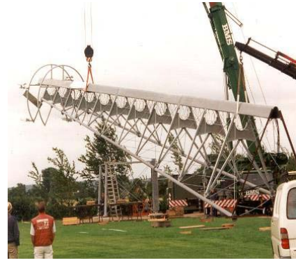
Fig. 19: Erection of the ID-Tower
