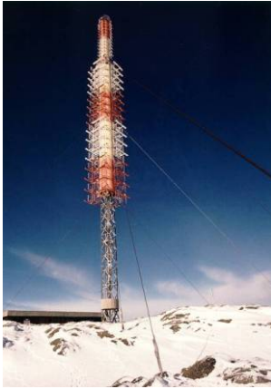
Fig. 9: Some masts are so heavily equipped with antennas so the wind resistance of the structure itself is not so important
