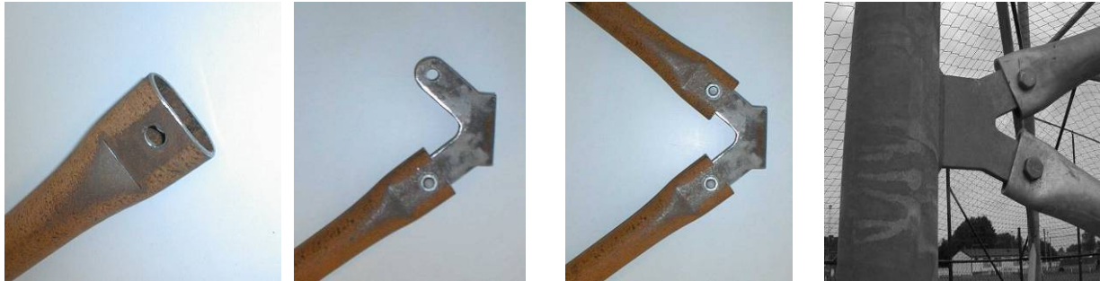
Figure 13: Principles of the assembly of the diagonals
