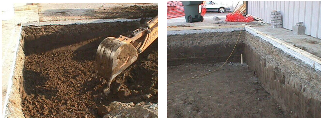
Image 5: a) Digging the hole for the base with a backhoe b) The hole is finished with straight and even edges.
