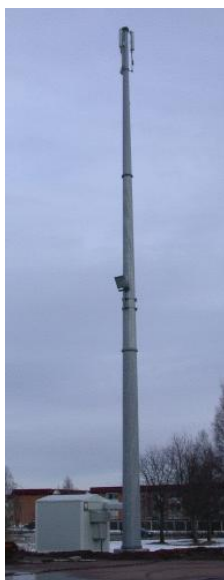
Image 2: A monopole tower Source: http://commons.wikimedia.org
