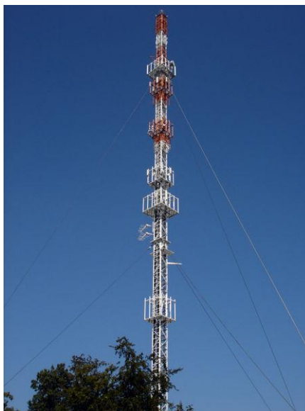
Image 14: A guyed mast with a total of six guy wires (two levels with 3 guys each).
