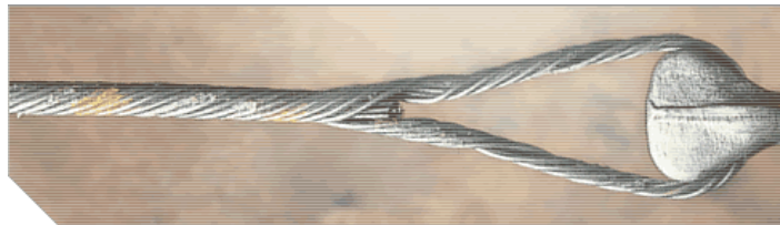
Image 12: A terminated guy cable with a "dead end".
