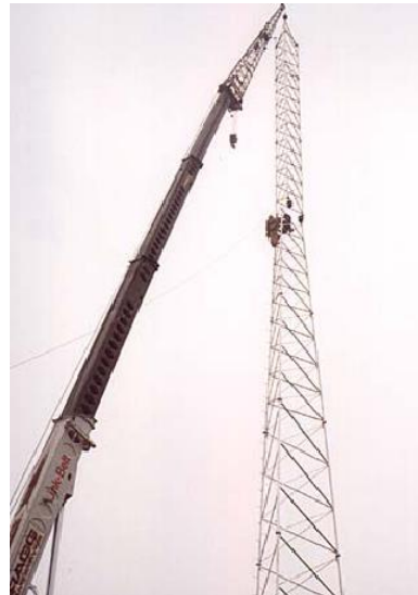
Image 9: Using a crane to place the top segment on a high self-supporting tower.
